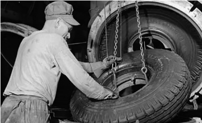
Workman removes a synthetic rubber tire from the vulcanizing oven at the Dominion Rubber plant. (Credit: Harry Rowed / National Film Board of Canada)
